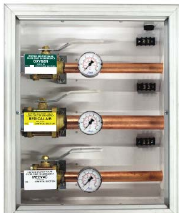
Zone Valve Boxes
